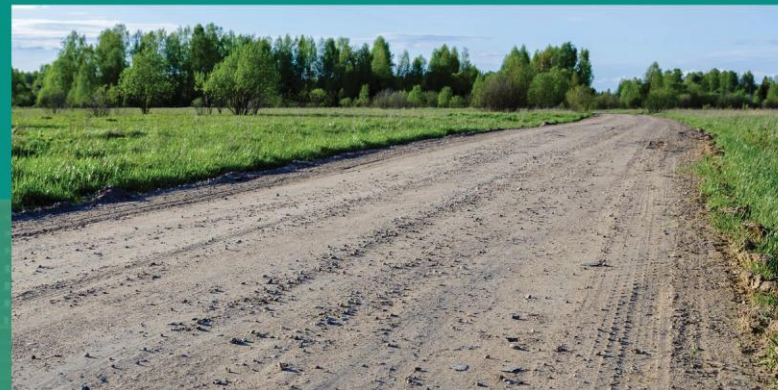
Temporary Agricultural Roads
